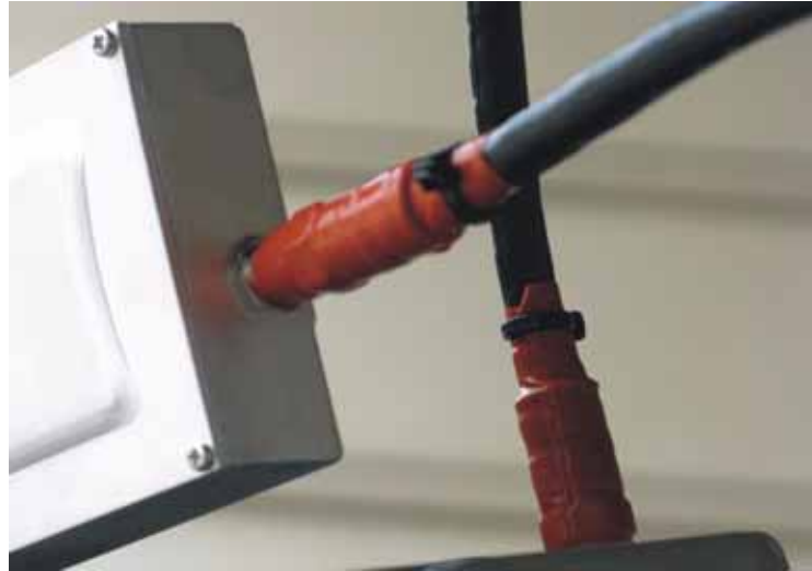
Figure 30: Weatherproofing the cable connectors
