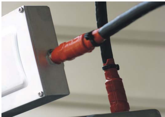
Figure 30: Weatherproofing the cable connectors
