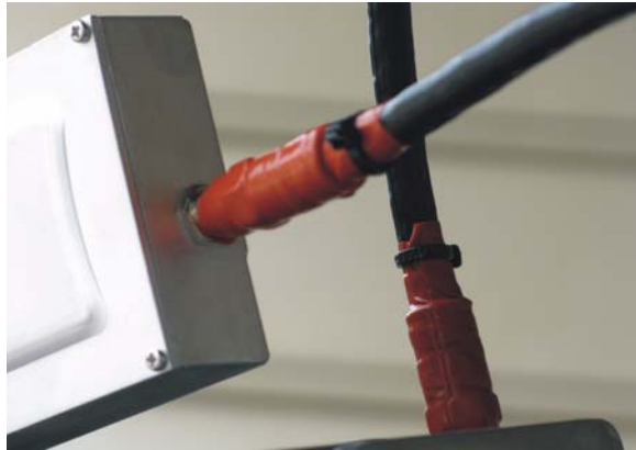
Figure 27: Weatherproofing the cable connectors
