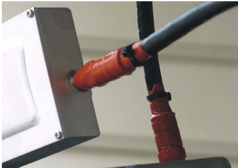
Figure 12: Weatherproofing the cable connectors
