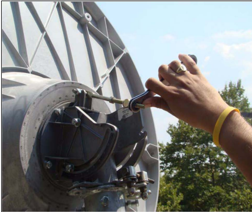
Installer adjusting elevation using fine EL tool
